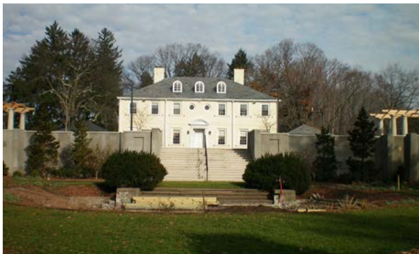
Greenwood Gardens recently completed its grant-funded project to restore its main terrace and garden steps. Read more about completed projects on page 15.
